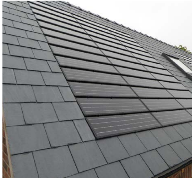
Figure 290: Contemporary solar panel design integrated within a traditional roofscape.
