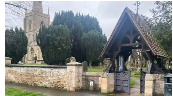
Figure 09: The Grade II* Listed Church of St Botolph in Quarrington.
