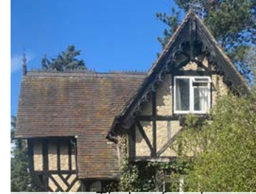
Figure 149: Timber framing.
