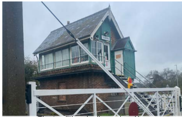
Figure 239: The traditional railway signal box.
