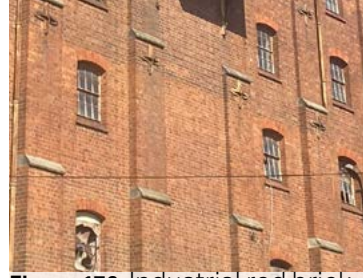
Figure 176: Industrial red brick.
