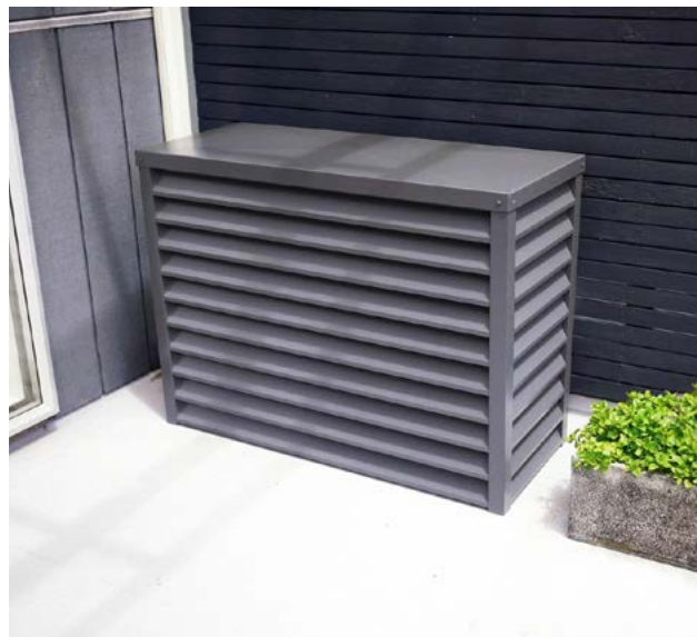
Figure 296: Air source heat pump housing covers the unit and harmonises with the building aesthetic.
