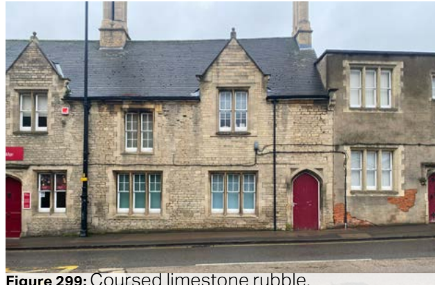
Figure 299: Coursed limestone rubble.
