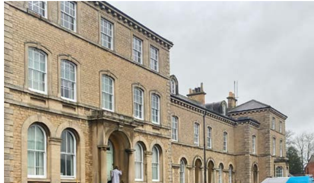
Figure 37: The landmark Grade II Listed Lafford Terrace.
