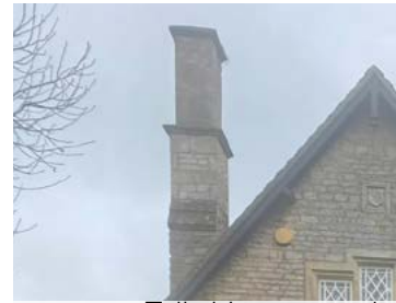
Figure 247: Tall chimney stacks.
