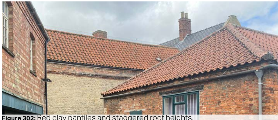
Figure 302: Red clay pantiles and staggered roof heights.
