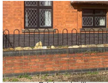
Figure 188: Brick and railings.
