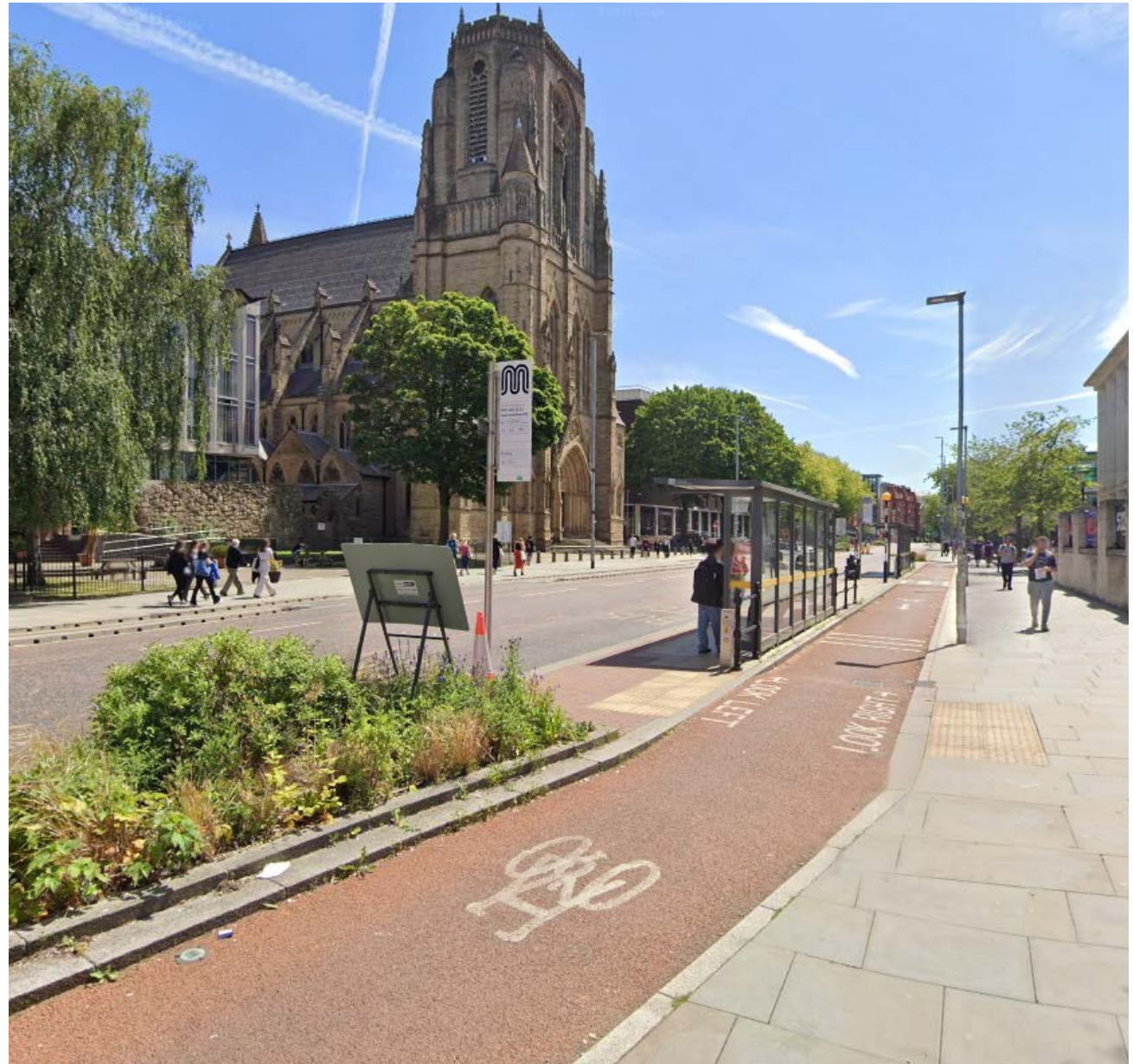
Figure 321: A cycle lane in Manchester in a defined colour and material, segregated from the carriageway by planting and not disrupted by the location of the bus shelter.
