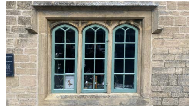
Figure 41: Neo-tudor stone window surrounds on a coursed limestone building.
