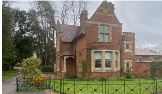
Figure 237: Red brick and stone surrounds are characteristic of the area.
