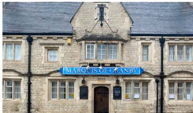
Figure 46: The Grade II Listed Marquis of Granby Public House (18th Century).
