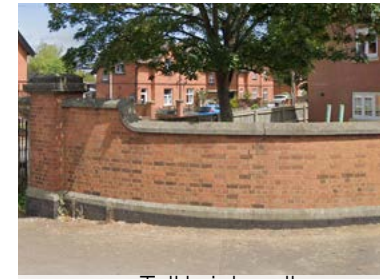
Figure 190: Tall brick wall.
