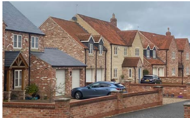
Figure 24: 21st Century housing along Mareham Lane.
