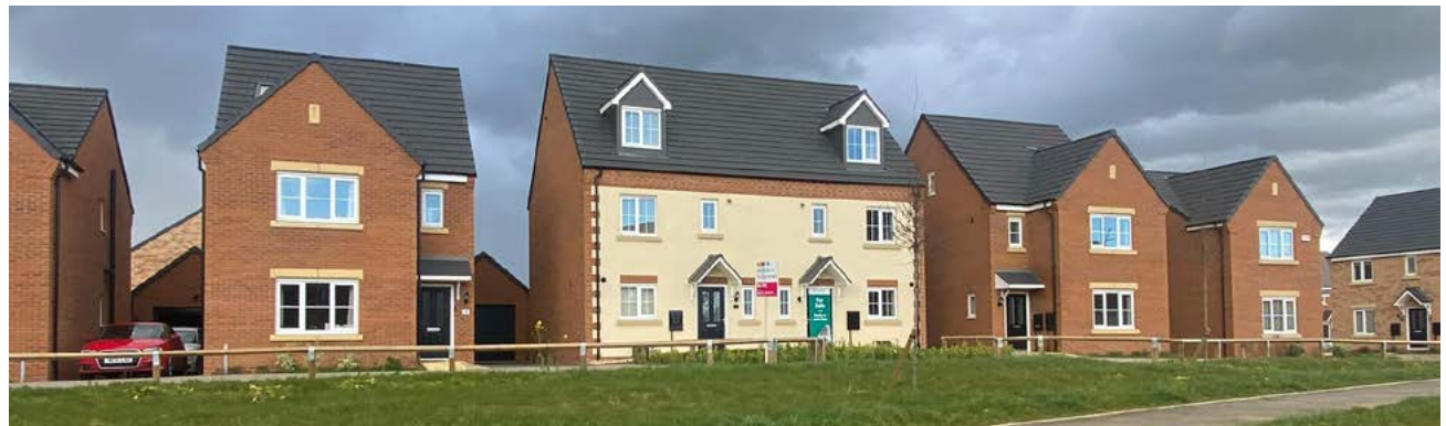
Figure 72: New homes along Whittle Road at NK/SLEA/002.
