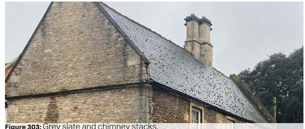
Figure 303: Grey slate and chimney stacks.
