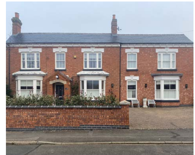
Figure 322: An extension in Leicestershire (right) that matches the existing dwelling in proportions, style and building materials with a slight difference in set-back to indicate the separate elements.
