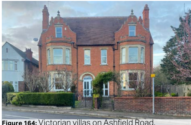
Figure 164: Victorian villas on Ashfield Road.
